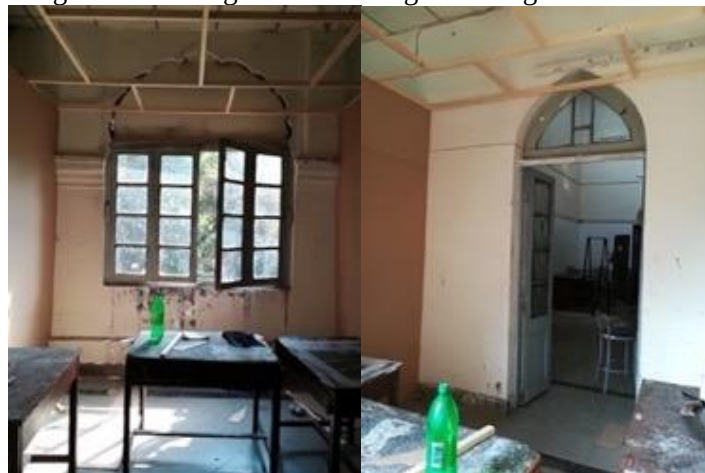
Left and right: making of panels ceiling and entrance, wood and lasani (wood)
