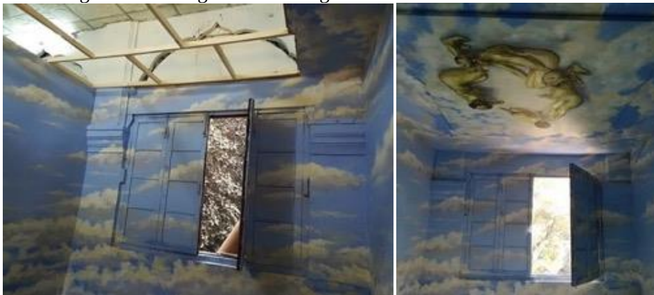
Left to right: ceiling before and after incorporation of 6x6 feet canvas
